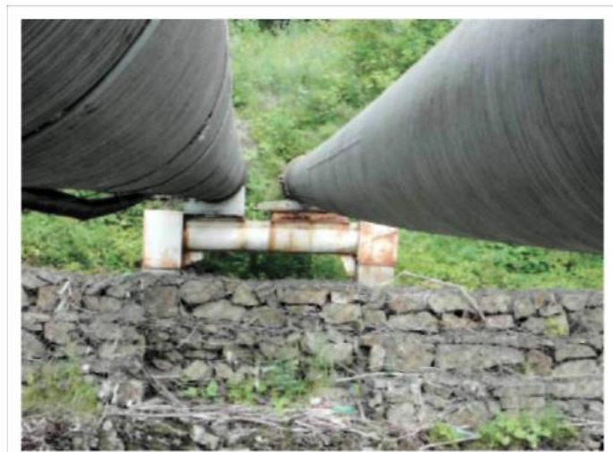
Fig. 3. Overall view of of the first (along the oil flow) bearing after repair.
